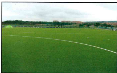
Work underway on the synthetic turf hockey field at Curro Hazeldean School in Pretoria
